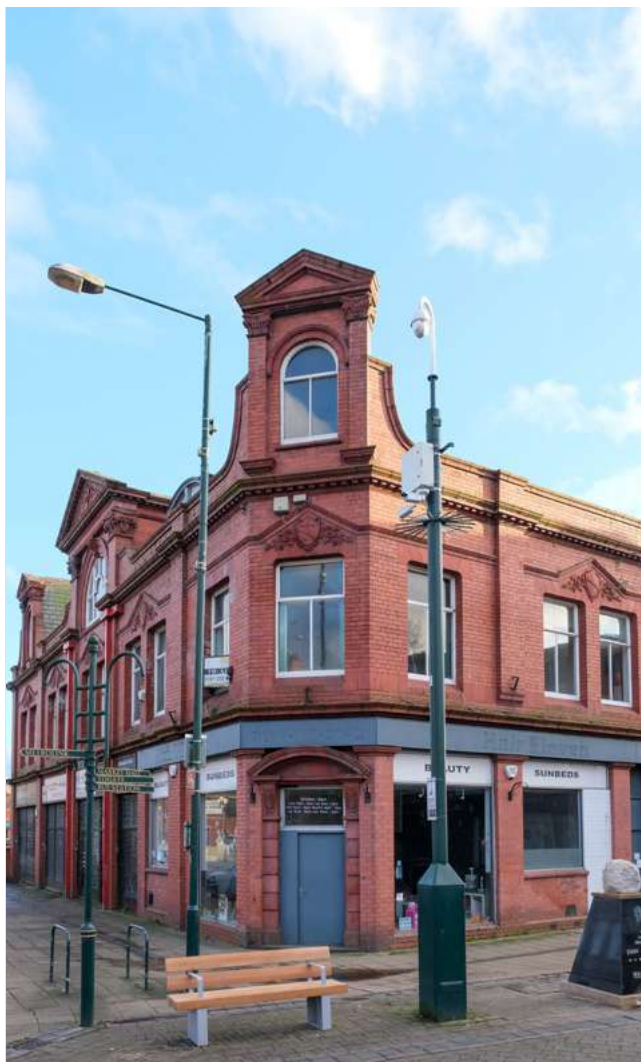
Market Chambers - a vacant Architectural Gem
